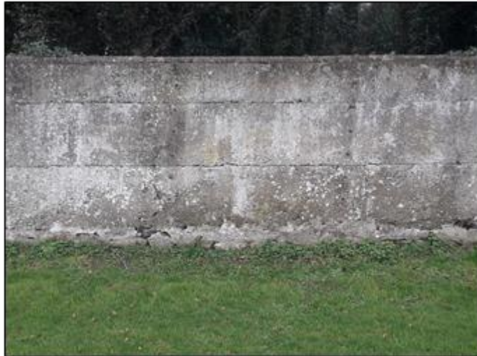
Plate 14.06: Looking east at boundary wall
